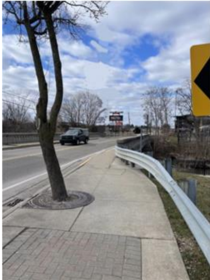
Figure 67: Light Pole Impeding Sidewalk Over Bridge After
