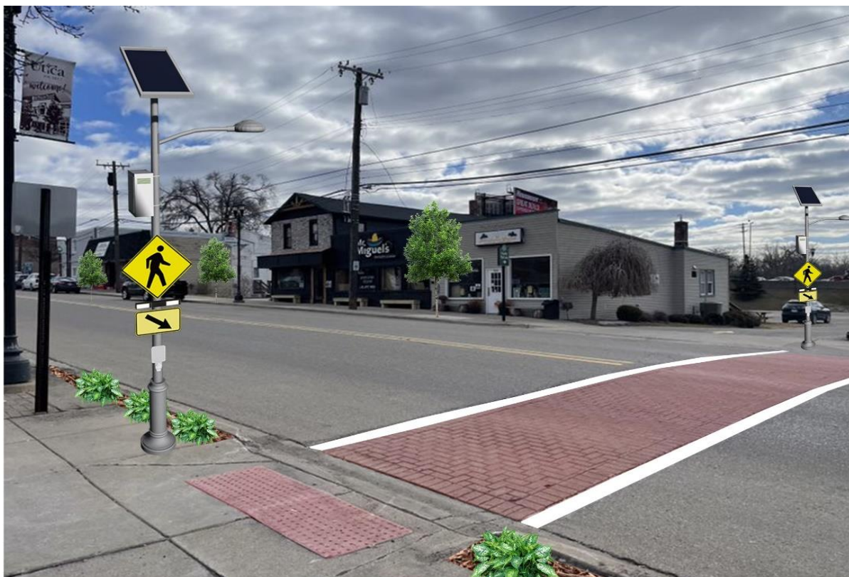
Figure 86: Auburn Road Crosswalk in front of Fire Station After
