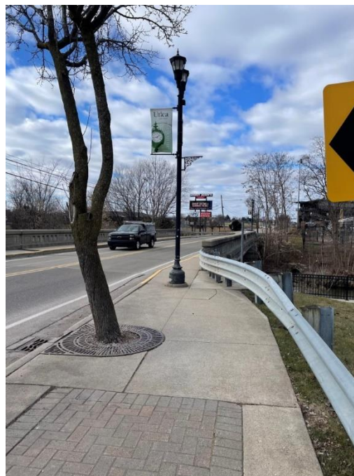
Figure 55: Auburn Road Bridge Over Clinton River Facing W; N Side of Auburn
