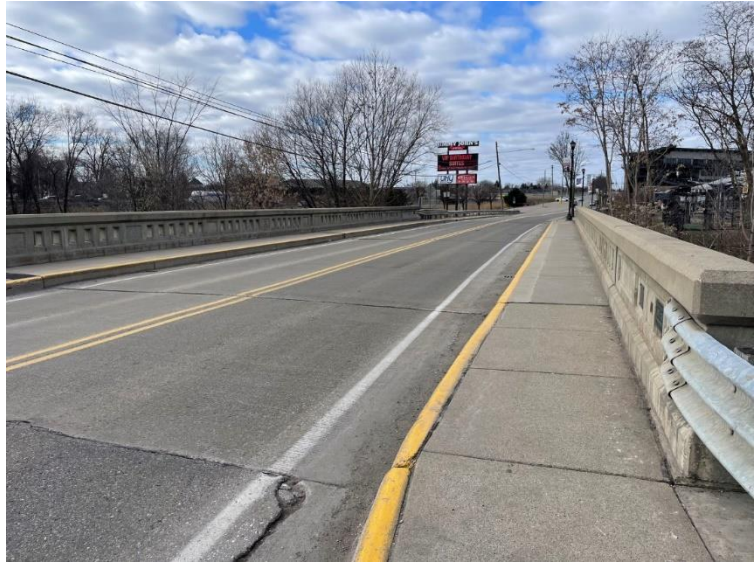
Figure 53: Auburn Road Over Clinton River Facing W; N Side of Auburn
