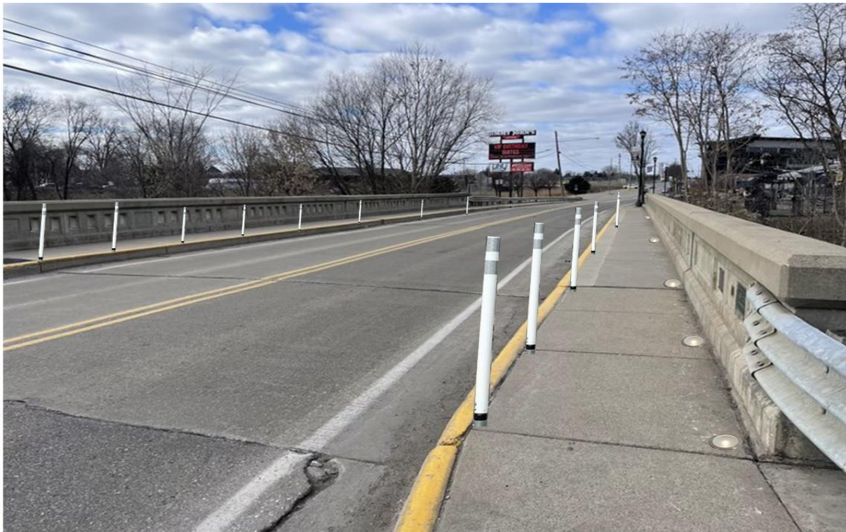
Figure 69: Bridge Over Clinton River After
