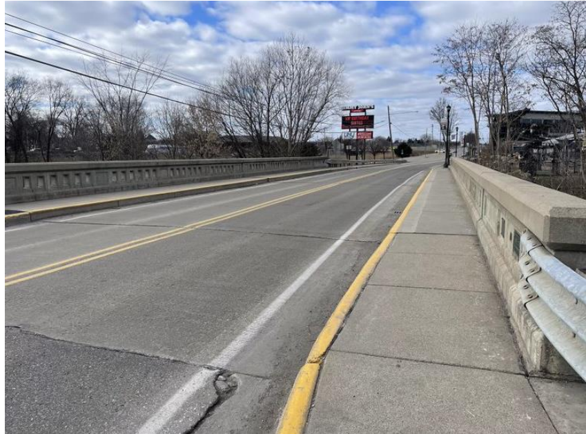
Figure 70: Bridge Over Clinton River Before
