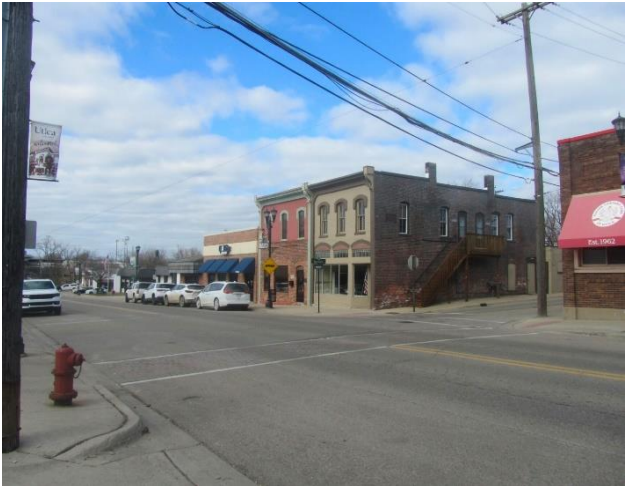
Figure 46: Auburn Road Facing W; S Side of Auburn
