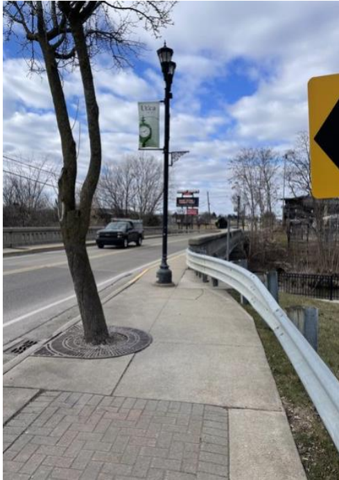
Figure 68: Light Pole Impeding Sidewalk Over Bridge Before
